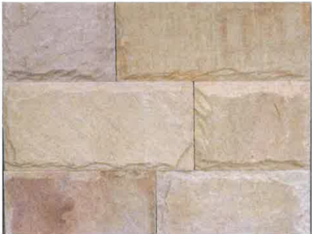
Code: EW4 Material: Sandstone Cladding, Rectangular Location: Lower Ground Floor Plinth (carparking level)
