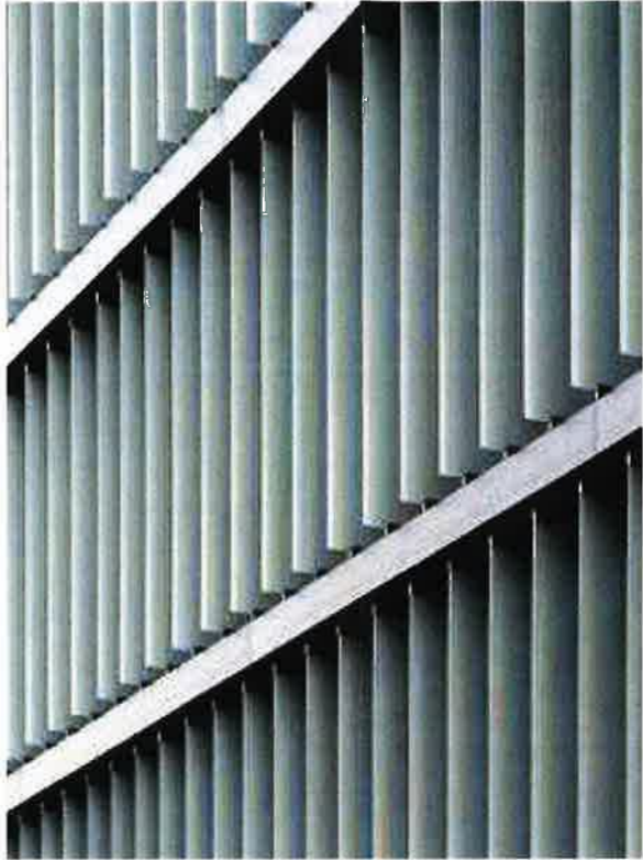
Code: EW3 Material: Aluminium Louvres, Colour to match Zinc Location: Lower Ground Floor Carpark
