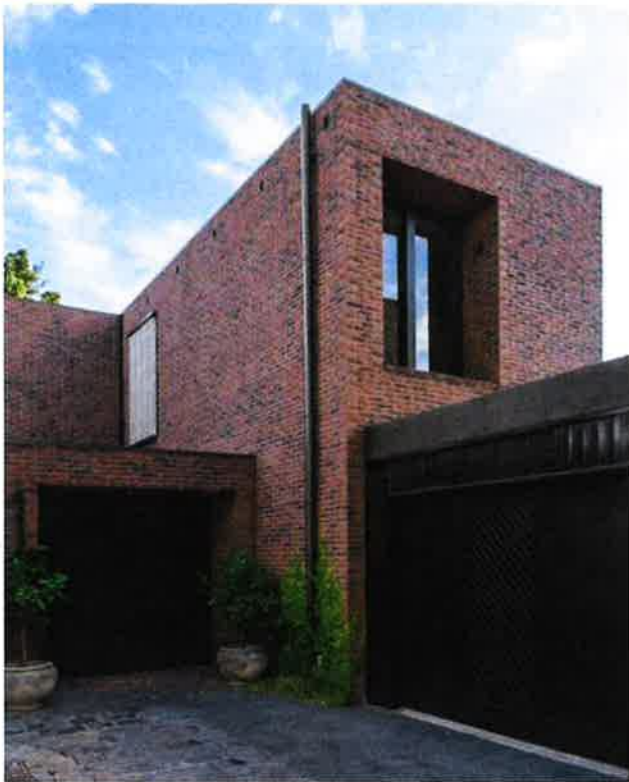
Code: EW1 Material: Red Brick- To match existing house. Pattern: Stretcher Bond laying pattern. Location: Walls Generally
