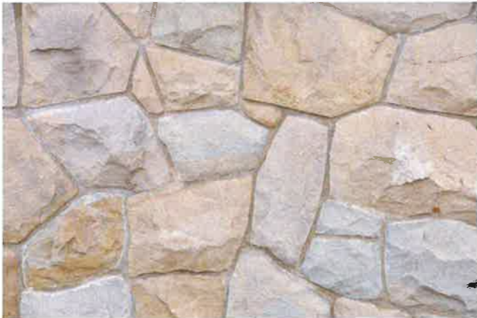
Code: EW5 Material: Existing Loose Sandstone Retaining Wall Disassembled and Rebuilt with Mortar To Form Lower Part of Plinth Location:
