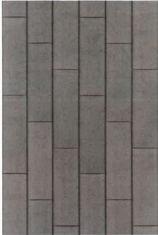
Code: EW2 Material: Grey metal cladding (Zinc or similar), Standing-seam or recessed joint vertical profiles Location: External Walls
